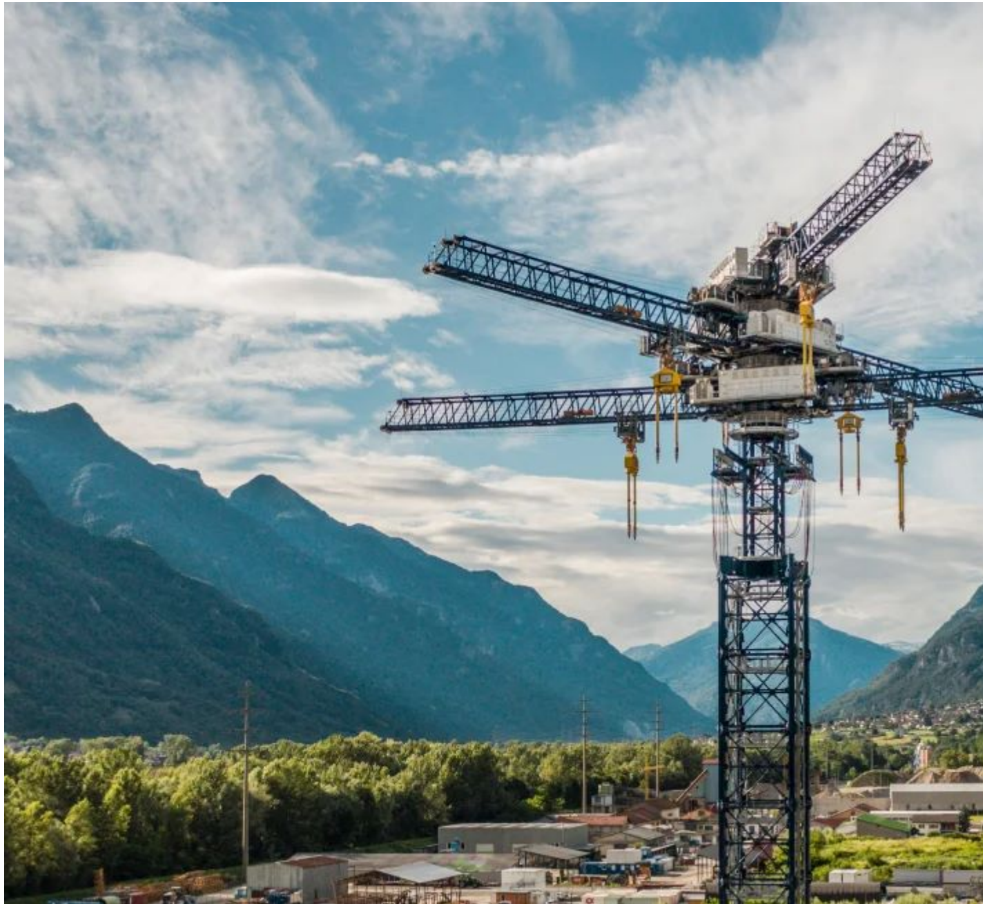
©Energy Vault Gravity storage
