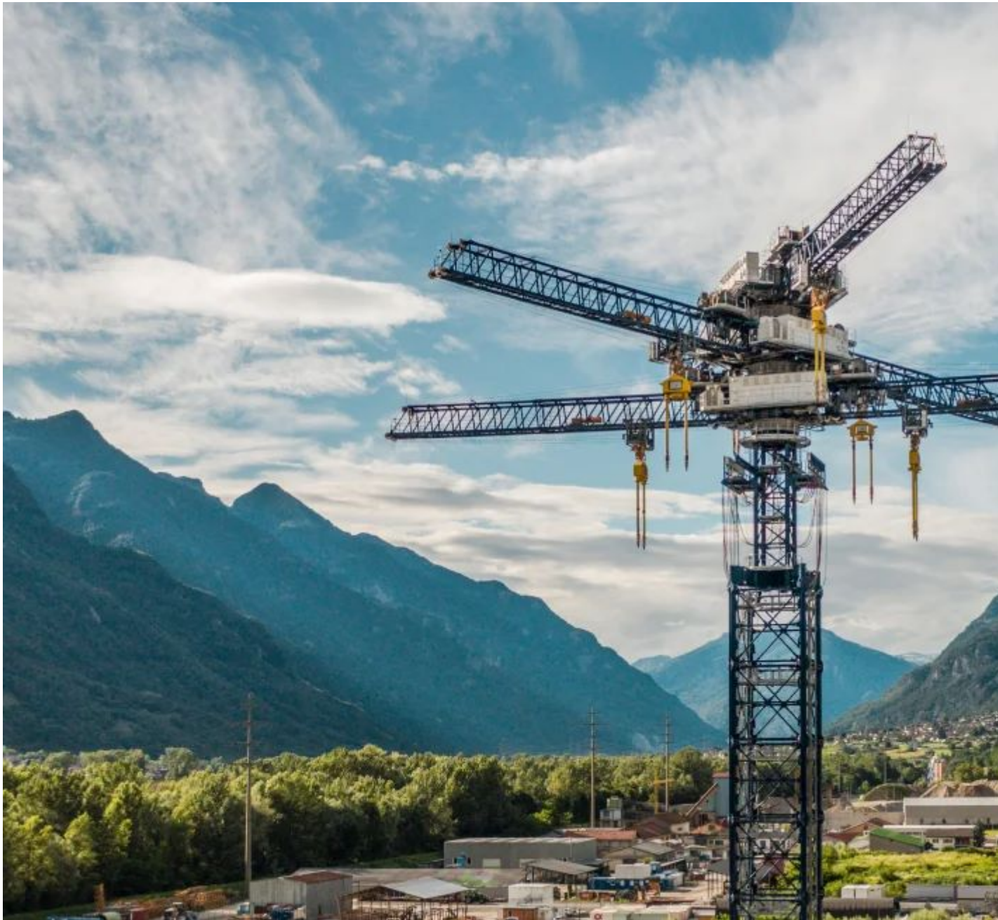
©Energy Vault Gravity storage
